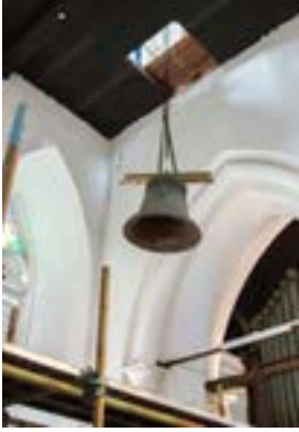
Lowering the bells down to the organ loft where they are lined up for a crane to take them out through a loft window.
