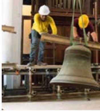
Lowering the bells down to the organ loft where they are lined up for a crane to take them out through a loft window.
