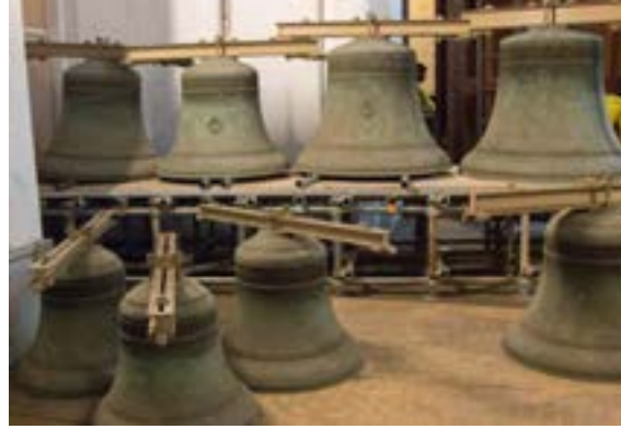
Lowering the bells down to the organ loft where they are lined up for a crane to take them out through a loft window.
