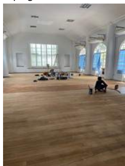
Polishing of NT Hall floor in progress
