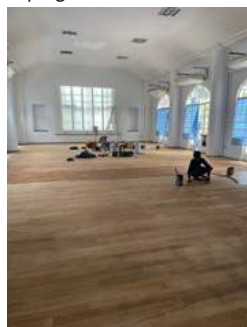
Polishing of NT Hall floor in progress
