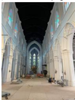
Scaffold removed. Lighting and fans installation in progress.
