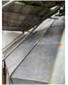
Lead sheet installation at apse
