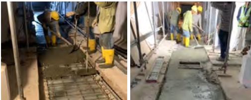
Trench casting works
