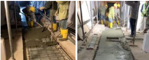
Trench casting works
