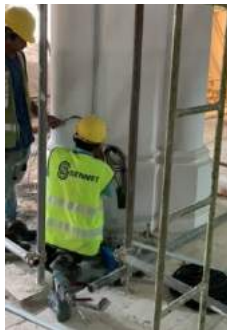
Cabling works in the Nave
