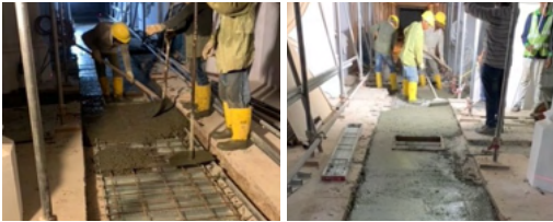
Trench casting works
