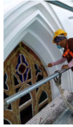
Application of wood preservatives
