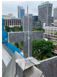
Leaded cross restored
