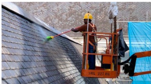
Washing of NT Roof slates in progress.
