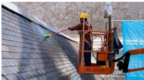
Washing of NT Roof slates in progress.
