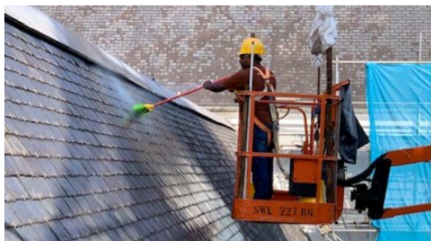
Washing of NT Roof slates in progress.
