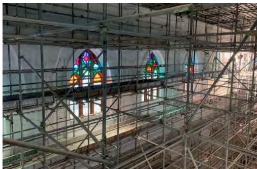
Plastering to North Side of Nave completed. Painting has commenced.
