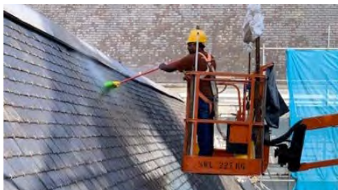
Washing of NT Roof slates in progress.
