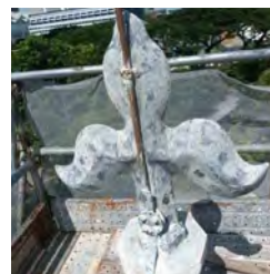
Existing fleur-de-lis above the sacristy, covered in lead sheet
