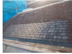
Trial wash to existing roof slates above South Transept
