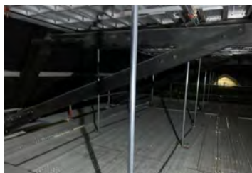
Inspection of nave's roof's truss
