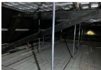
Inspection of nave's roof's truss
