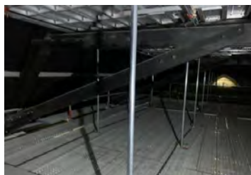
Inspection of nave's roof's truss
