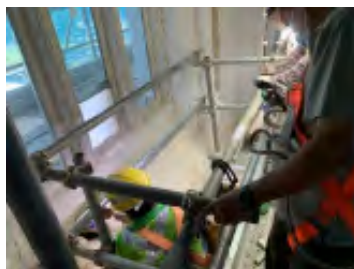
Repairs to cracks being carried out at the South Clerestory
