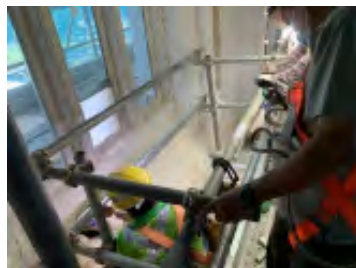
Repairs to cracks being carried out at the South Clerestory
