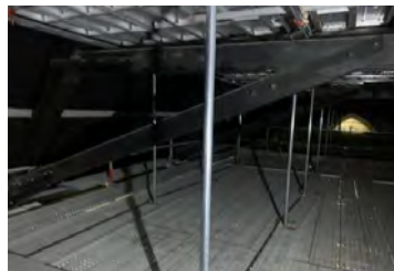
Inspection of nave's roof's truss
