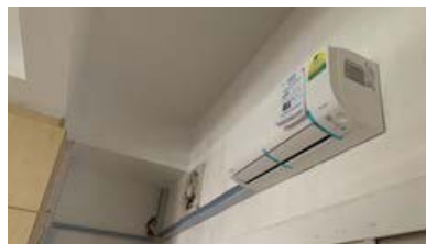
Air con installation at Graham White Library
