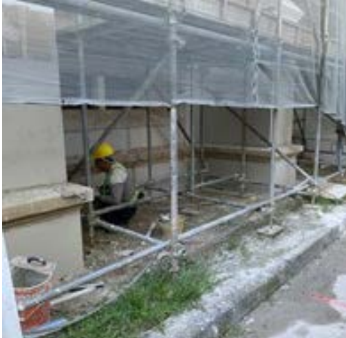
Plastering works outside South side of Nave
