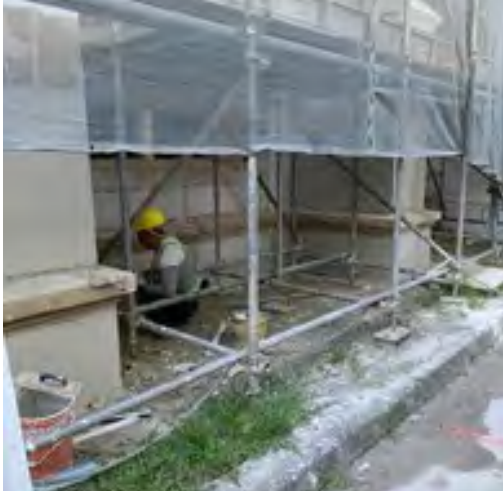
Plastering works outside South side of Nave
