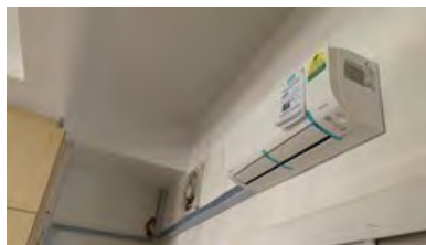
Air con installation at Graham White Library
