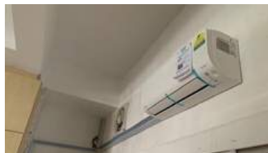
Air con installation at Graham White Library
