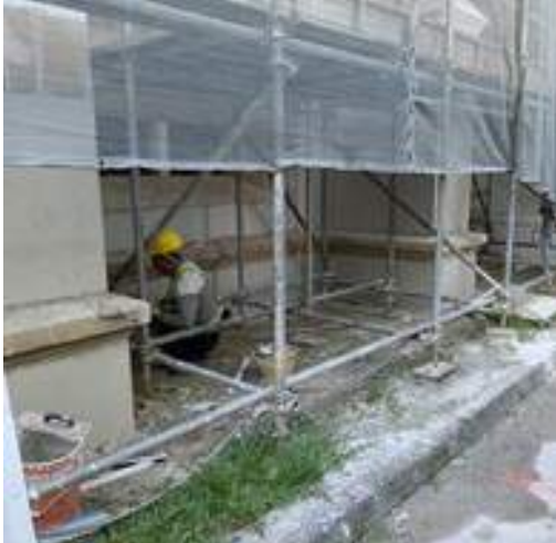
Plastering works outside South side of Nave
