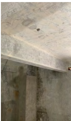
Removal of paint at L2 South Transept
