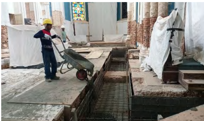
Casting of reinforced concrete at trenches
