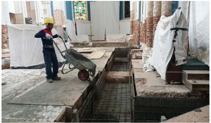
Casting of reinforced concrete at trenches
