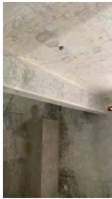
Removal of paint at L2 South Transept
