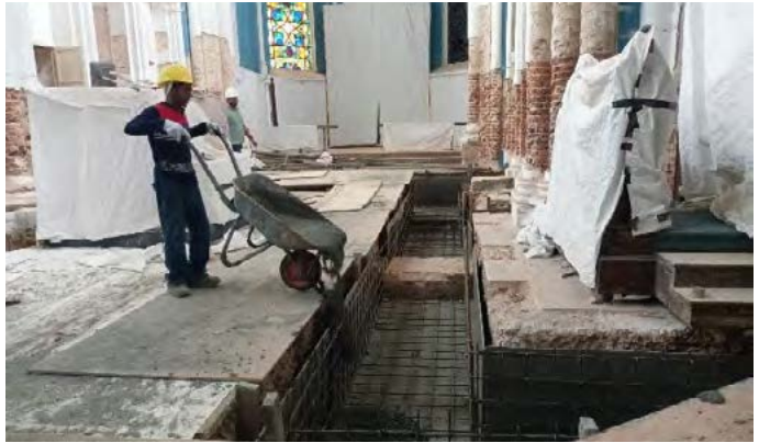
Casting of reinforced concrete at trenches
