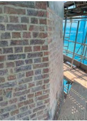
Removal of cement plaster from external walls at bell tower
