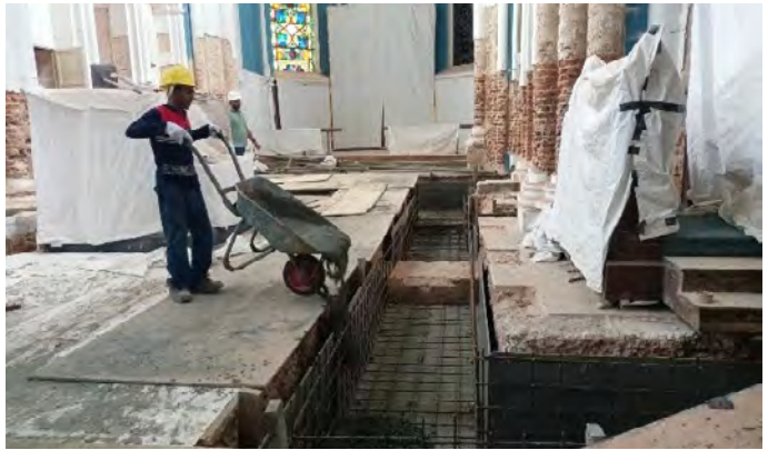
Casting of reinforced concrete at trenches
