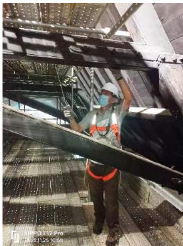
Inspection of nave's roof truss and timber
