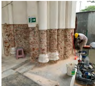
Top: Scaffold from South side reaching East side Left: Removal of wall plaster at West Porch Right: Bricks surface preparation works
