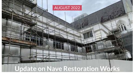
We continue to praise and thank God for the consistent number of workers on the site. Most of the workers are now deployed externally. The plaster removal at the North side is nearing completion. We can expect similar works to continue on the South side next week. Bricks surface preparations have commenced at the East and North
