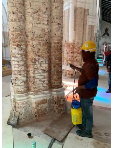
Biocide treatment on exposed wall of bricks
