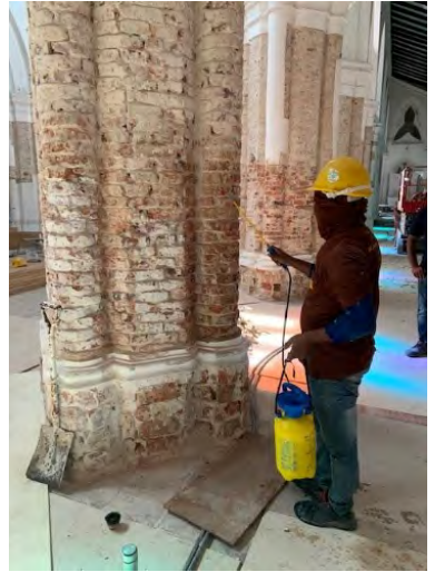
Biocide treatment on exposed wall of bricks
