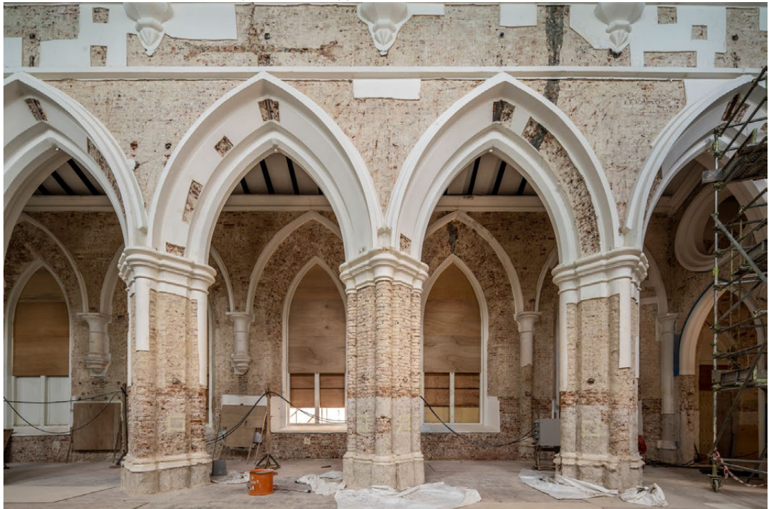
Crack lines caused during the building of City Hall MRT Station next to the Cathedral were discovered after the removal of plaster at the upper level of the Nave.
