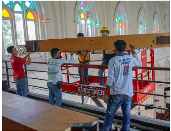
Reinstallation of wooden pipes at the gallery upon return from the UK.
