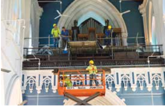
Workers removing the pipes by means of a scissor lift
